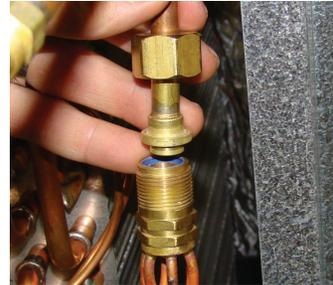
4. Slide the 13/16" nut over the lineset and separate the two halves of the flowrator.
