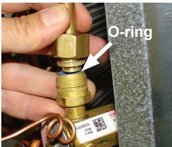
**III-6.** Remove the additional Teflon O-ring seal from the box and place on the shoulder just inside the TXV inlet port. Screw the nut attached to the liquid line portion of the flowrator body onto the inlet port of the TXV.
