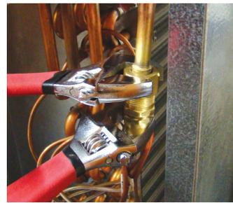
3. After ensuring that the coil is free of any residual pressure, disassemble the flowrator body completely using two wrenches. Take great care not to distort the feeder tubes. The wrench used to clasp the nut should be turned in counter-clockwise direction to unscrew the nut.
