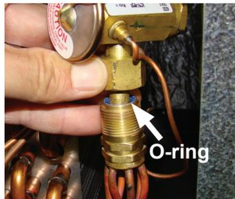
**III-5.** After ensuring that the Teflon O-ring seal is still in place inside the flowrator body, screw the female swivel nut onto the flowrator body.
